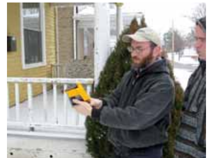
Weatherization Inspector Ted Ramp uses an infrared camera to show Chris the areas of greatest energy loss in the house.
